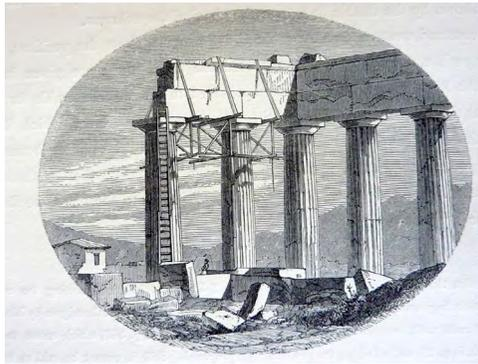
Figure 21.13. Measuring the deviations from the orthogonal of the Parthenon columns. Engraved vignette in Penrose's book.<sup>65</sup>
