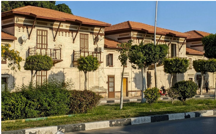
Fig. 11.3 SCC workers' villas in Port Fouad. Author's photograph, 2020, CC BY-NC-ND.
