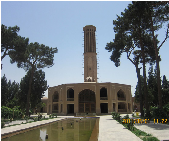
Fig. 9.5 Dolatabad pavilion: natural ventilation is carried out through the wind catcher. Yazd, Iran. Author's photograph, 2011, CC BY-NC-ND.
