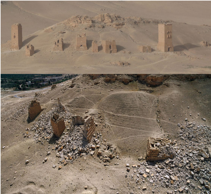
Fig. 2.6 Six tower tombs. Damage assesment of Palmyra. Photographs by DGAM, 2017, CC BY-NC-ND.
