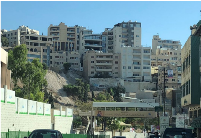
Fig. 4.5 Recent residential constructions blocking the view of Bsharat Church in Lweibdeh. Author's photograph, 2020, CC BY-NC-ND.
