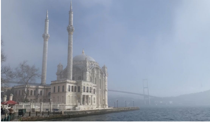
Fig. 12.1 Ortaköy Mosque or Grand Imperial Mosque of Sultan Abdümejid designed in the Neo-Baroque style as an example of a unique atmospheric architectural masterpiece with a distinctive view of the Bosphorus Strait and Bridge connecting the European and Asian parts of the city. Author's photograph, 2021, CC BY-NC-ND.
