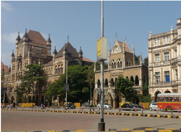
Fig. 1.2 Examples of buildings in Victorian Gothic architecture—Elphinstone College, David Sassoon Library and Army Navy Building (Kala Ghoda). Author's photograph, 2018, CC BY-NC-ND.
