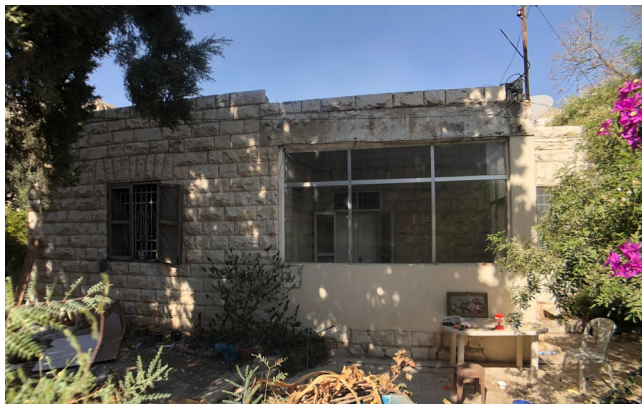
Fig. 4.3 The vacant House C in Lweibdeh. Author’s photograph, 2020, CC BY-NC-ND.
